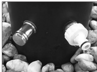
Discharge opening with a drain plug (left), inlet fitting with hose connector (right)
